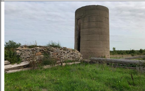
IMAGE 15 SILO AND BARN FOUNDATION
