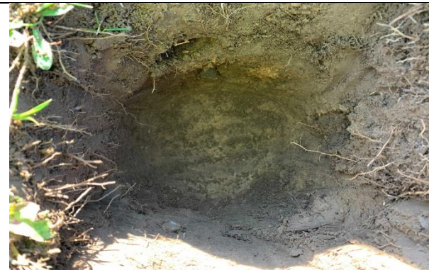
IMAGE 16 TEST PIT IN PROGRESS
